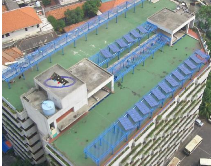
Figure 8. The PV grid connected on the BPPT building.
